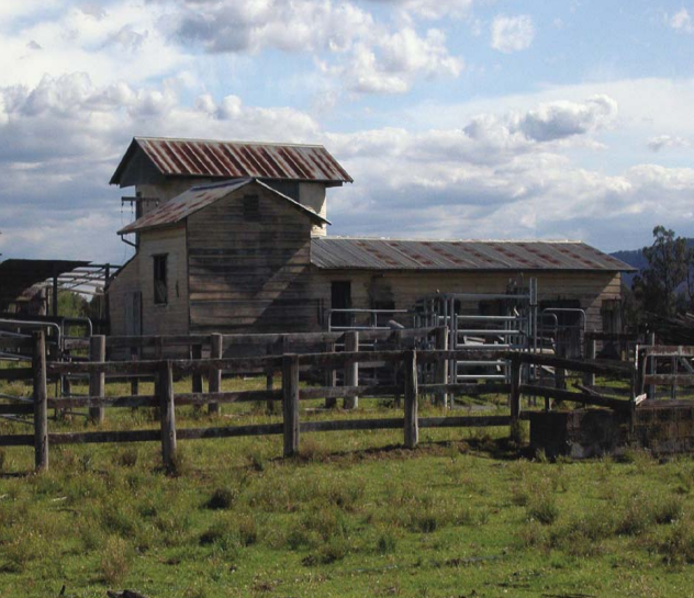
Example of old and new construction showing similar forms
