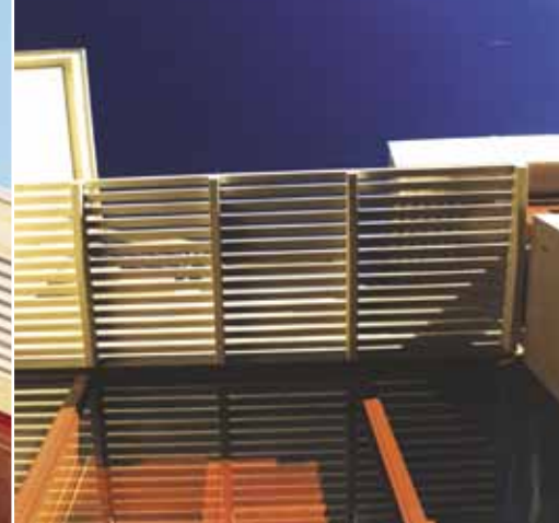
Horizontal timber slats offer a good alternative to solar protection and eave overhang.
